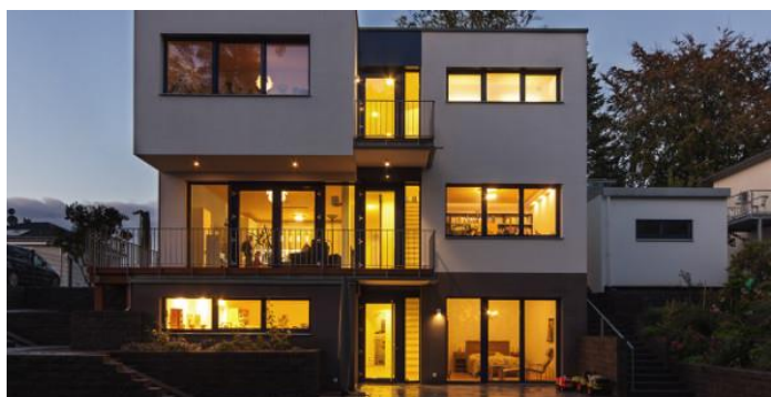
Passive House in Berlin with renewable energy and utilisation of rainwater. © Andrea Kroth
