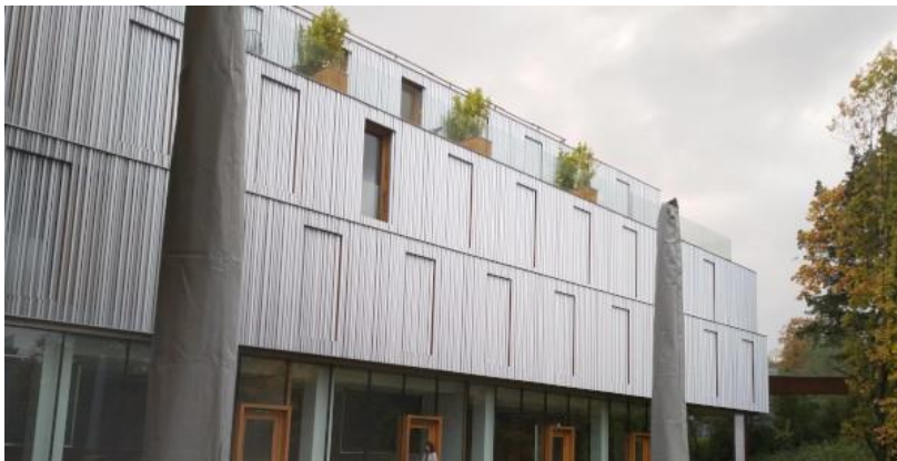
Eyecatching even in rainy weather. This Passive House hotel in the Spanish town of San Sebastián was built using a lot of wood and was on the itinerary of an excursion within the framework of the COP25 in Spain. © PHI
