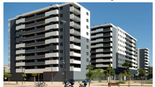
Social housing for 160 families in Saragossa, Spain. The four buildings are equipped with PV systems and are certified as Passive House Plus. © Grupo Lobe
