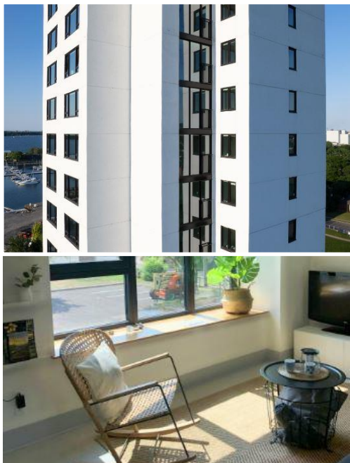
The 1960s Ken Soble Tower after retrofitting to the EnerPHit standard. © Courtesy Double Space & ERA Architects
